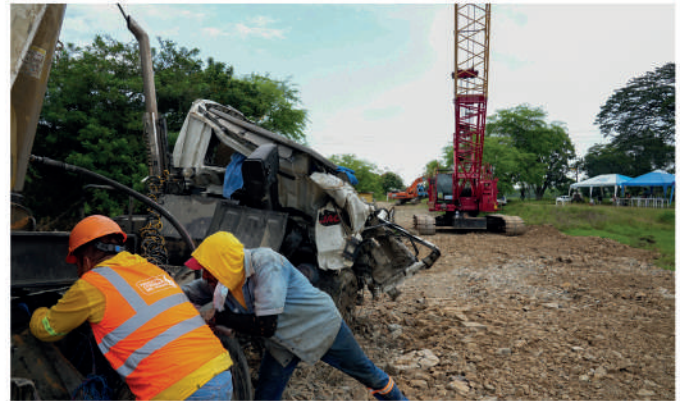
La Prefectura Ciudadana del Guayas, a través de la concesionaria, instaló maquinaria especializada. The Guayas Citizen Prefecture, through the concessionaire, installed specialized machinery.
